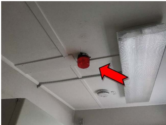
Photo 3. Interior, ground level, laundry room, ceiling – assumed asbestos-containing fibre cement sheeting.
