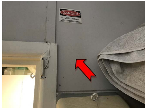
Photo 2. Interior, ground level, laundry room, wall – assumed asbestos-containing fibre cement sheeting.
